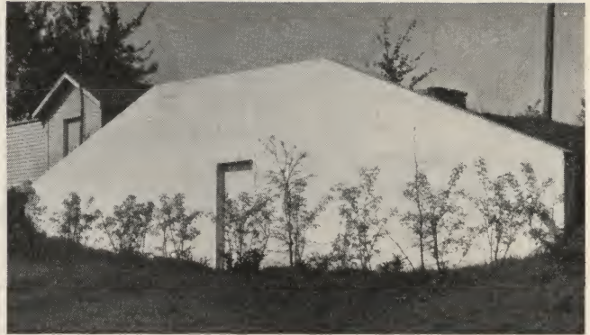
Home-grown fruit and vegetables can be kept in good condition for a considerable period of time when stored in an underground concrete storage cellar or cave.
